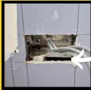
Pencil lines shown here are attempts from the dry-liner to cut around the back box on a party wall.
